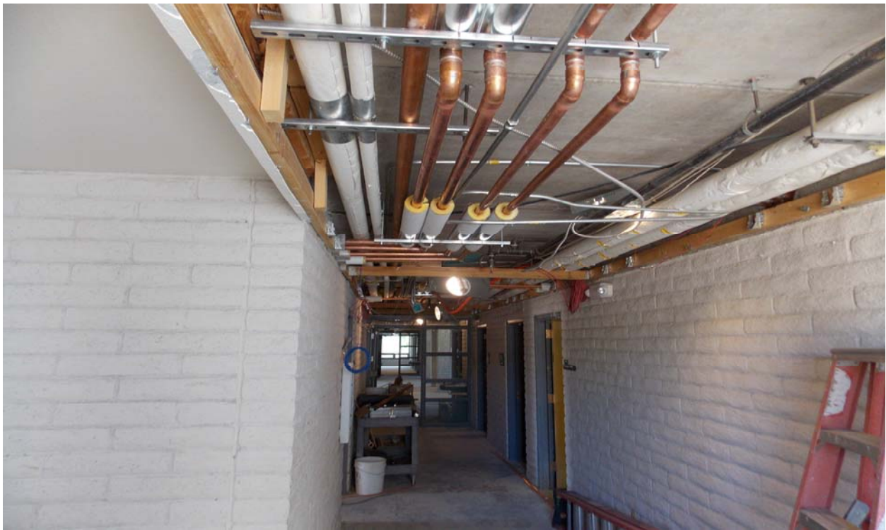
Installation of Piping for Room Heating and Cooling Units
