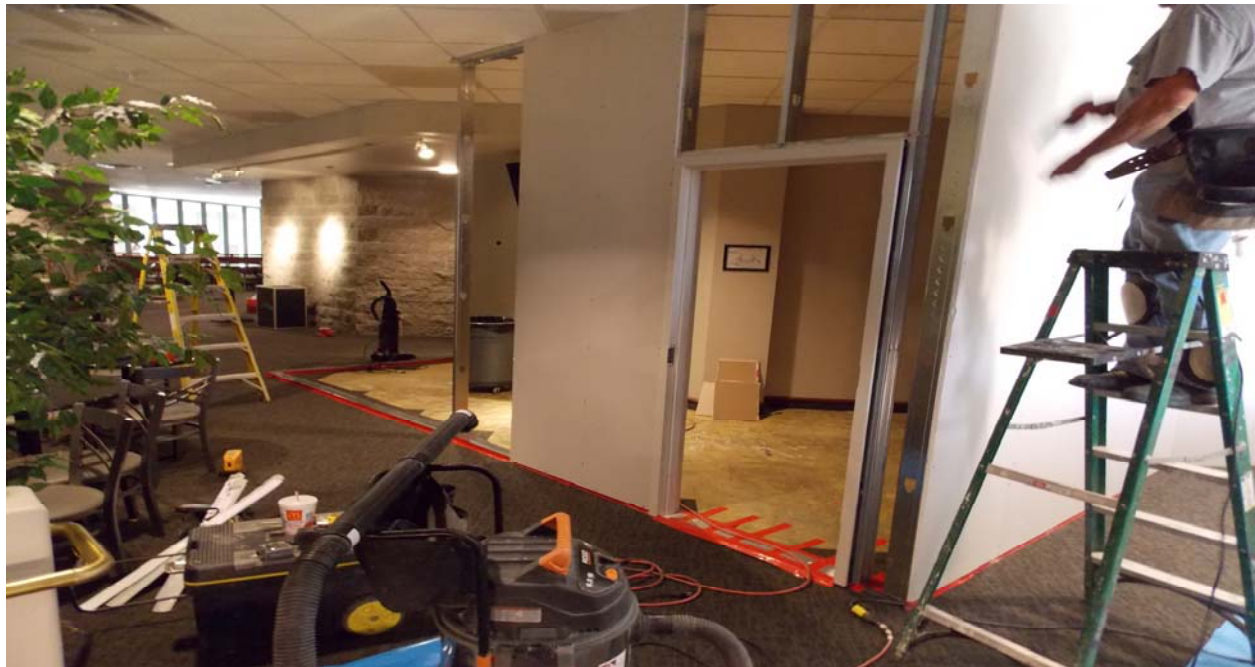
Framing of Serving Room 308A
