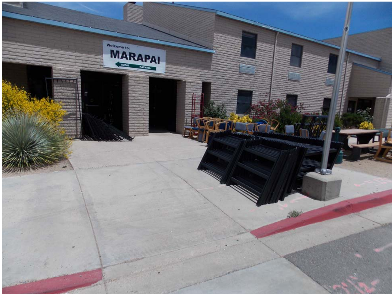
Furniture Removed from Marapai in Preparation for Construction
