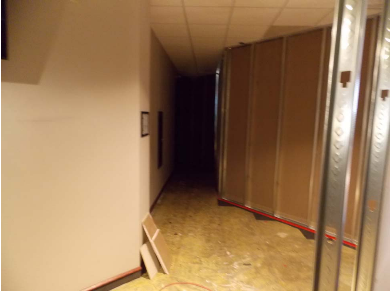
Framing of Serving Room 315
